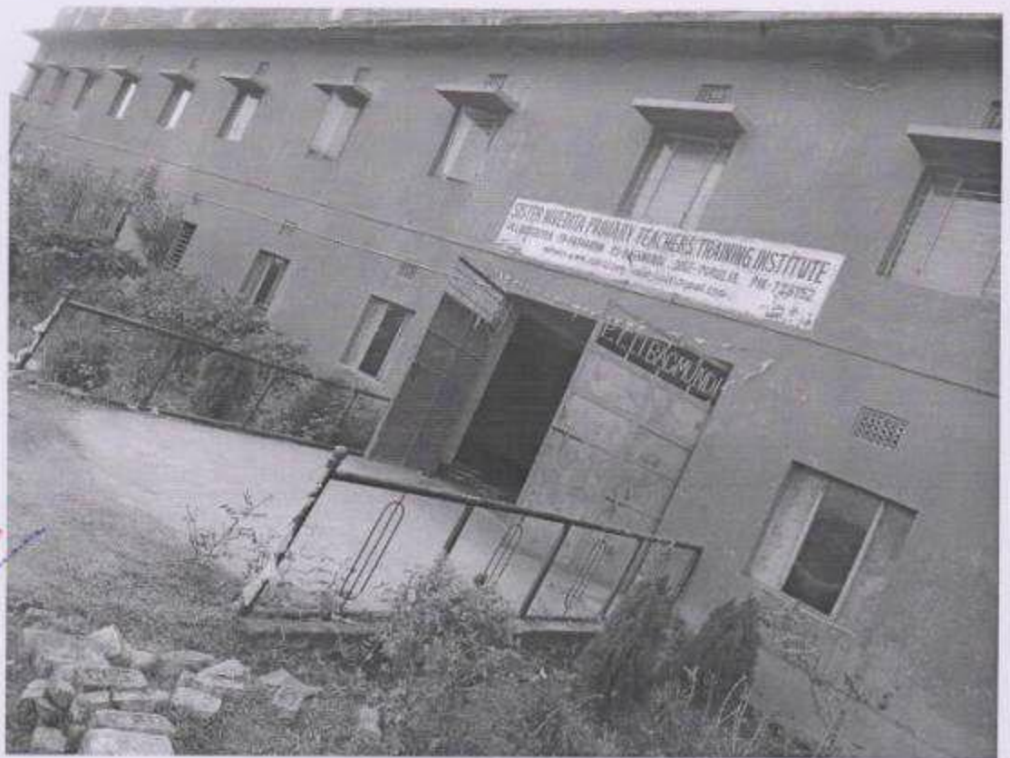
Front view of the Building
